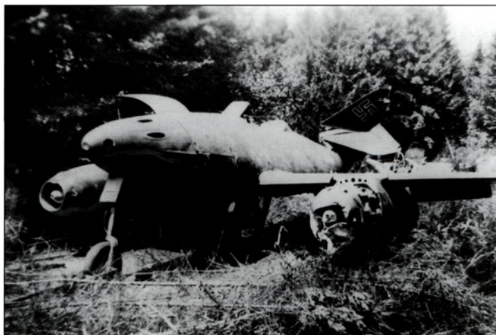
Not all of JV 44's Me 262s made it to Salzburg or Innsbruck. Here, Wk-Nr. 111074 is pictured abandoned in the Hofoldingen Forest. It appears as if the aircraft has been deliberately damaged with an explosive charge of some kind at the join between the fuselage and the tail assembly, and that the Jumo 004 engine nacelles have been damaged with a hammer, or been driven in to. Note that the nosewheel towbar has been left fixed to the wheel – evidence of hurried action
