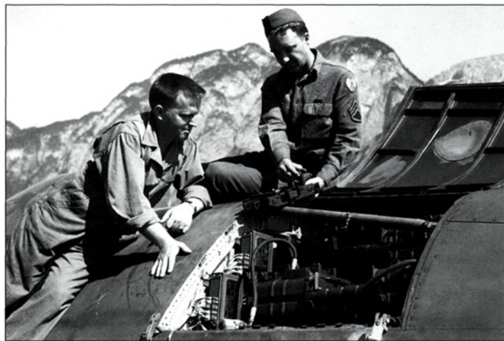
Armourers from the US Ninth Air Force enjoy an opportunity to inspect at first hand the ‘business end’ of an Me 262 of JV 44 at Innsbruck-Hötting shortly after the cessation of hostilities. Note the electric ignition cable attached to the lower 30 mm MK 108 cannon
