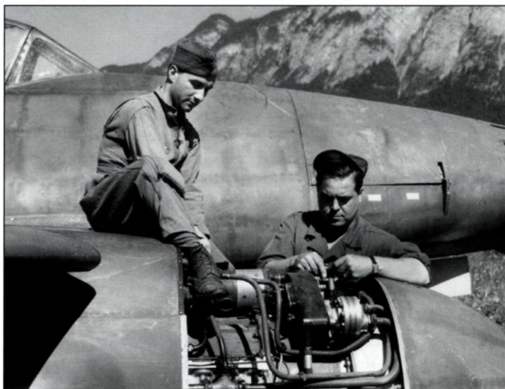
Engine technicians of the US Ninth Air Force inspect the Jumo 004 jet engine of an Me 262A-1a of JV 44 at Innsbruck in May 1945
